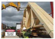
5. The operator must position the forklift in an appropriate area to ensure the trusses are lifted safely. The forklift will take the weight of the trusses on the forks ensuring no one is within the danger area.
