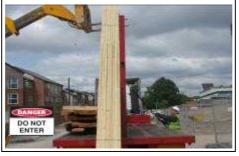
8. The forklift truck operator must lift the trusses from the trailer and then move the trusses to a safe and / or off-load area.
