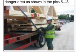
7. The driver will release the individual rope / banding attaching the pack to the bars. This must be carried out from a safe position.
