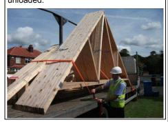
7. The driver will then separate each truss at the heel by placing a wedge between the first and second truss.
