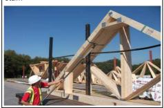
6. Once the load stability has been checked the driver will loosen the transportation straps on the side being unloaded.
