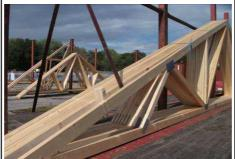
9. The customer team will then take hold of the truss while the driver cuts the blue rope. Once the blue rope has been cut the team will then off load the truss in a safe manner. Proceed with this recommended method for the remaining trusses.
