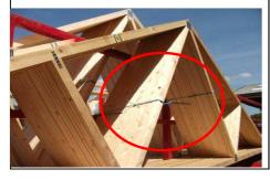
5. The driver will cut the **banding** securing the truss pack to allow separation of the individual trusses. This must be carried out using a closed blade pruning staff.
