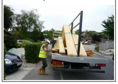
4. The manufacturer will supply truss packs secured to the trailer with blue 3 core rope / banding. You shall familiarise yourself with which rope attaches which pack to the centre bars.
