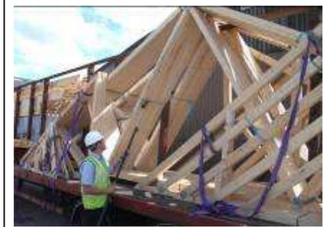
8. The crane will then lift the truss pack from the bed of the trailer. **NEVER** stand in the danger area where the trusses could potentially fall. Do not allow any others to enter the danger area.
