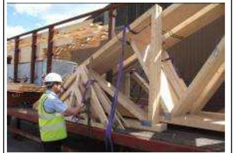
7. The driver will release the individual rope / banding attaching the pack to the bars. This must be carried out from a safe position.
