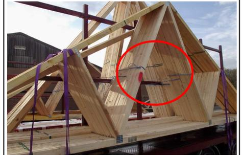
4. Once the order of unloading is agreed between the slinger and driver, the slinger will attach the purple lifting slings to the crane hooks.
