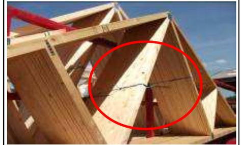
4. On instruction from the site responsible person the driver will release the transport straps on the side being unloaded ensuring no one is within the danger area as shown in the pics 5—8.
