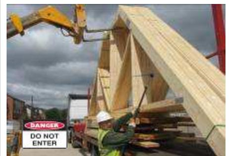
8. The forklift truck operator must lift the trusses from the trailer and then move the trusses to a safe and / or off-load area.
