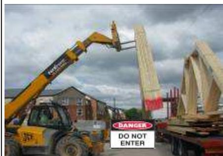
9. Other products are removed from the load as per applicable SSoW. Metalwork bags and straps must be removed from the trailer in conjunction with the drivers specific manual handling training.
