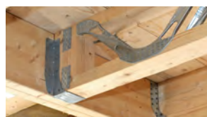
Cullen Universal Hanger, Gang-Nail plate and SpaceJoist metal web designed using Gang-Nail software.
